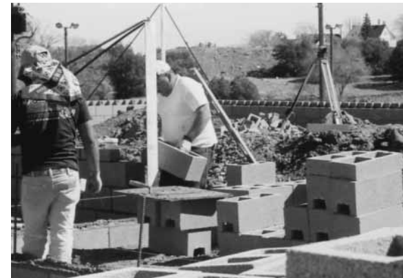
Ernie's crew onsite at Rusing Hills
